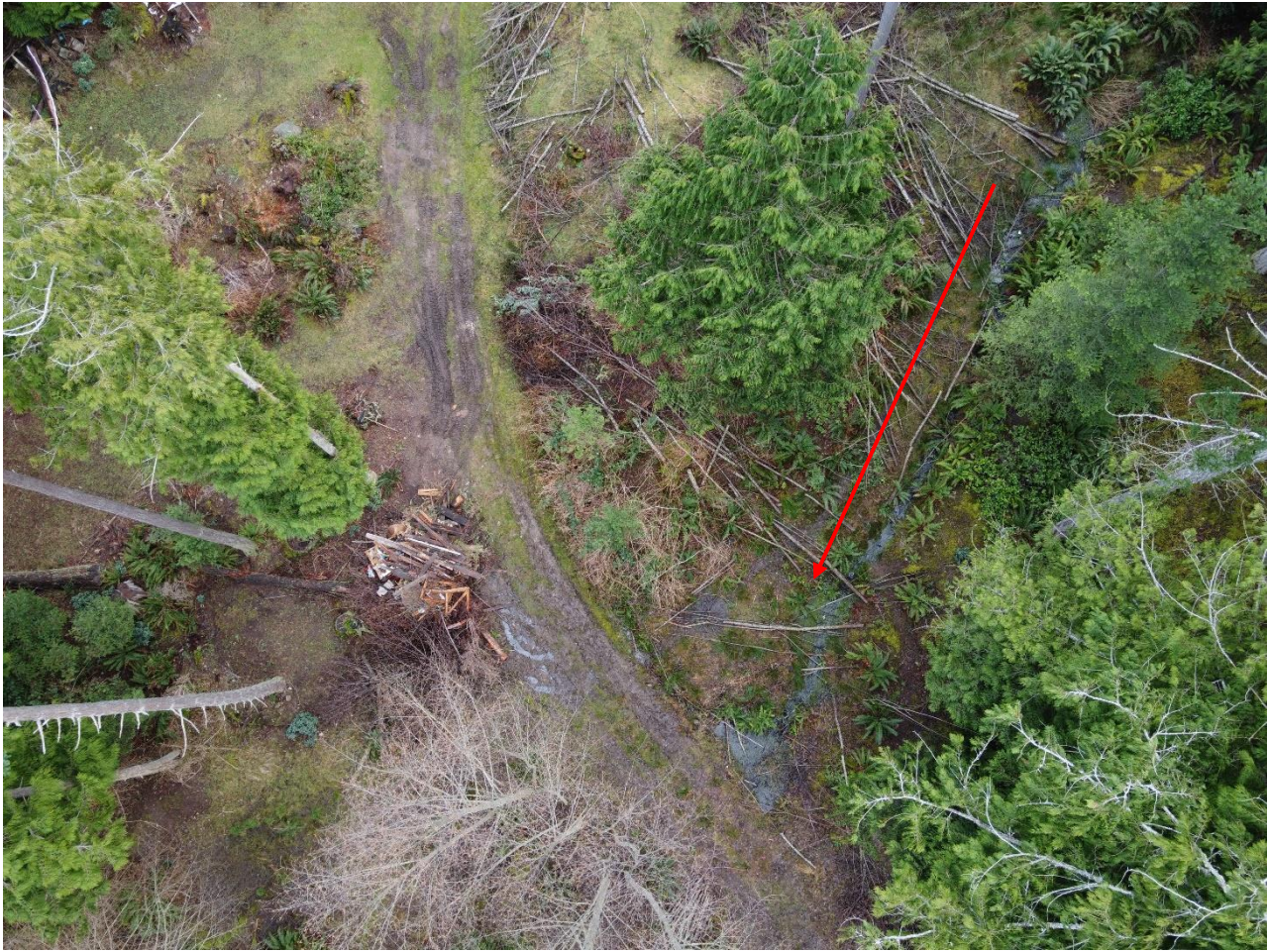
Figure 7. Old logging roads, compacted soil surfaces, and a deep ditch with flowing water (red arrow) could be removed to restore a forested cedar wetland in this location. The ditch concentrates and directs runoff onto the neighbouring properties to the north.
