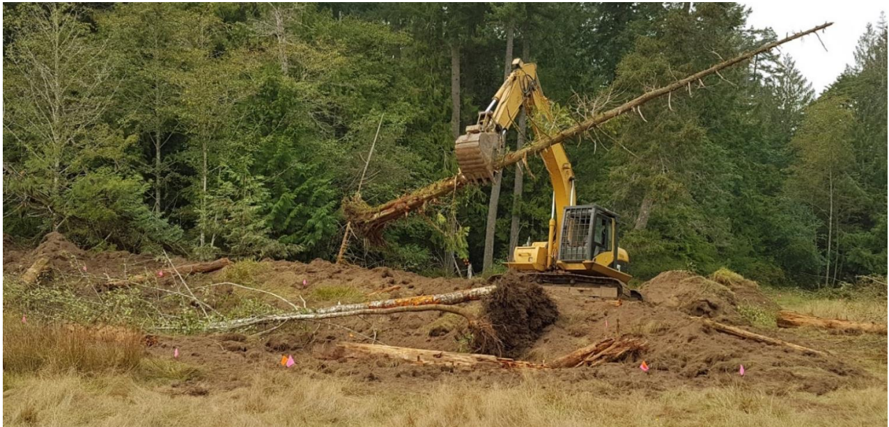
Figure 12 Adding coarse woody debris sourced on site to a wetland pond in September 2020 at Xwaaqw'um (Burgoyne Bay Provincial Park), Salt Spring Island.
